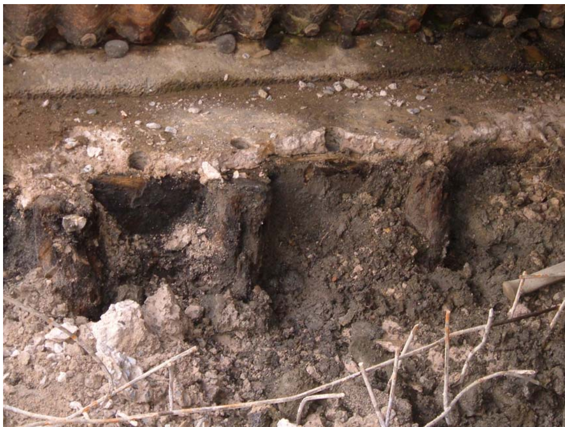
Plate 4: Close-up of timber pegs on west side of bridge arch, looking west
