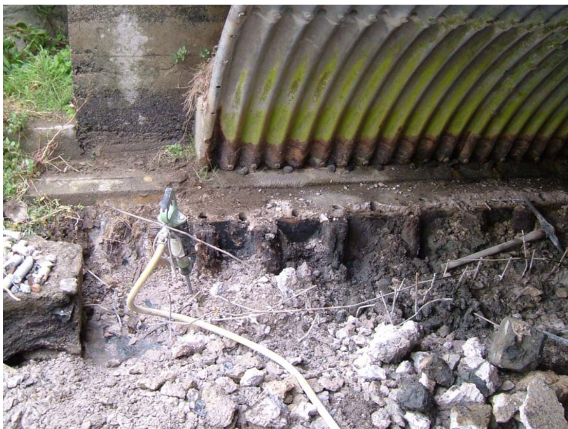
Plate 3: Exposed upright timber pegs on west side of bridge arch, looking west
