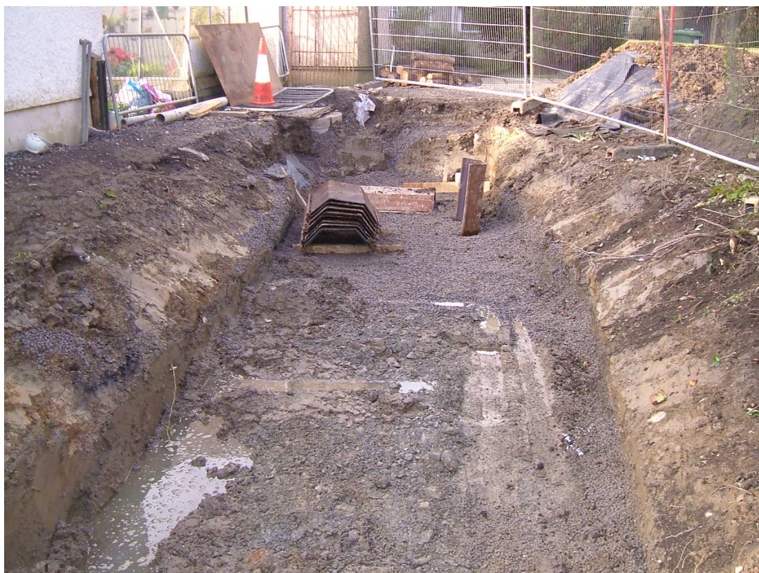
Plate 2: Excavation of flood wall footing, Island House
