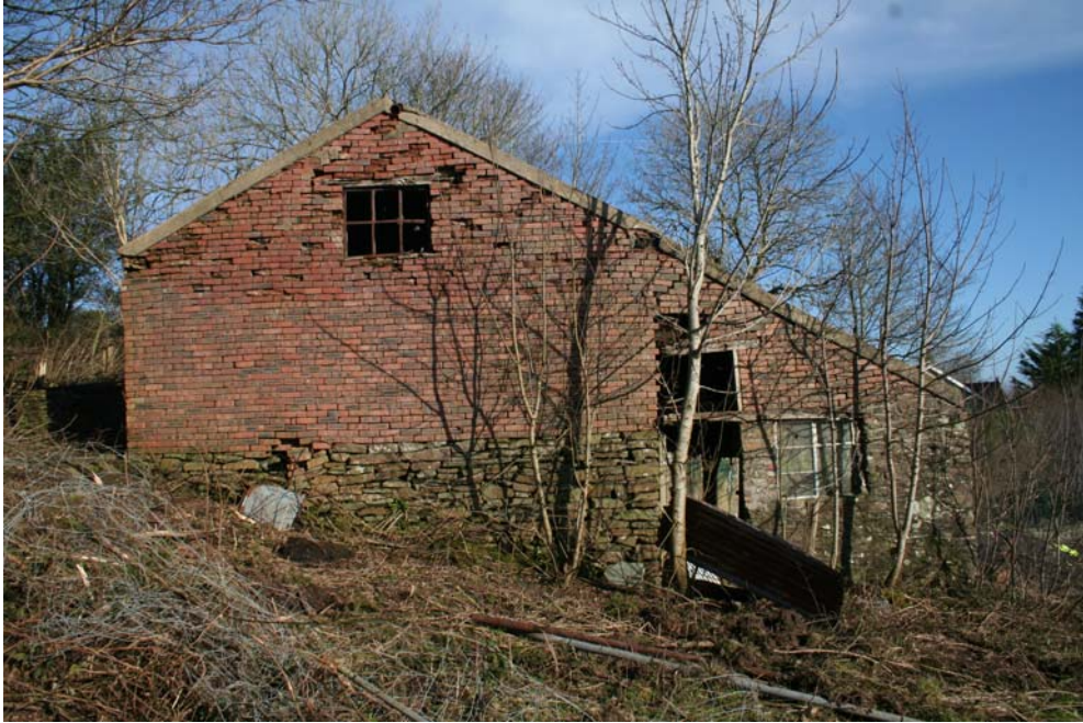
Plate 2: Gable end of existing building showing stone and brick construction.
