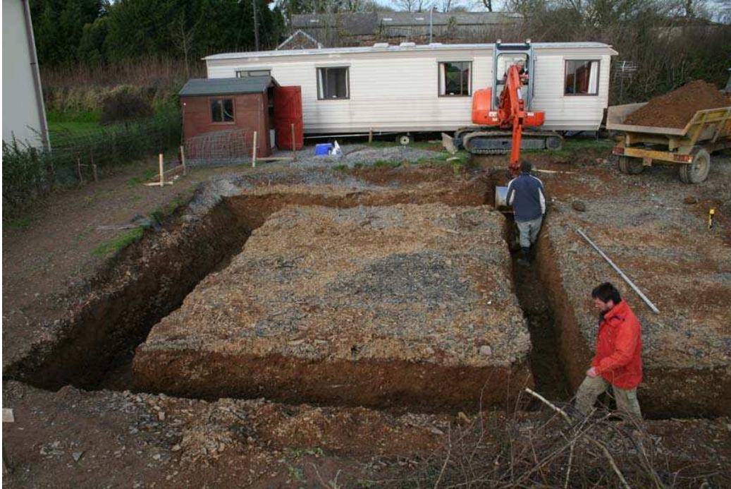
Plate 2: Excavation of foundation trenches in progress
