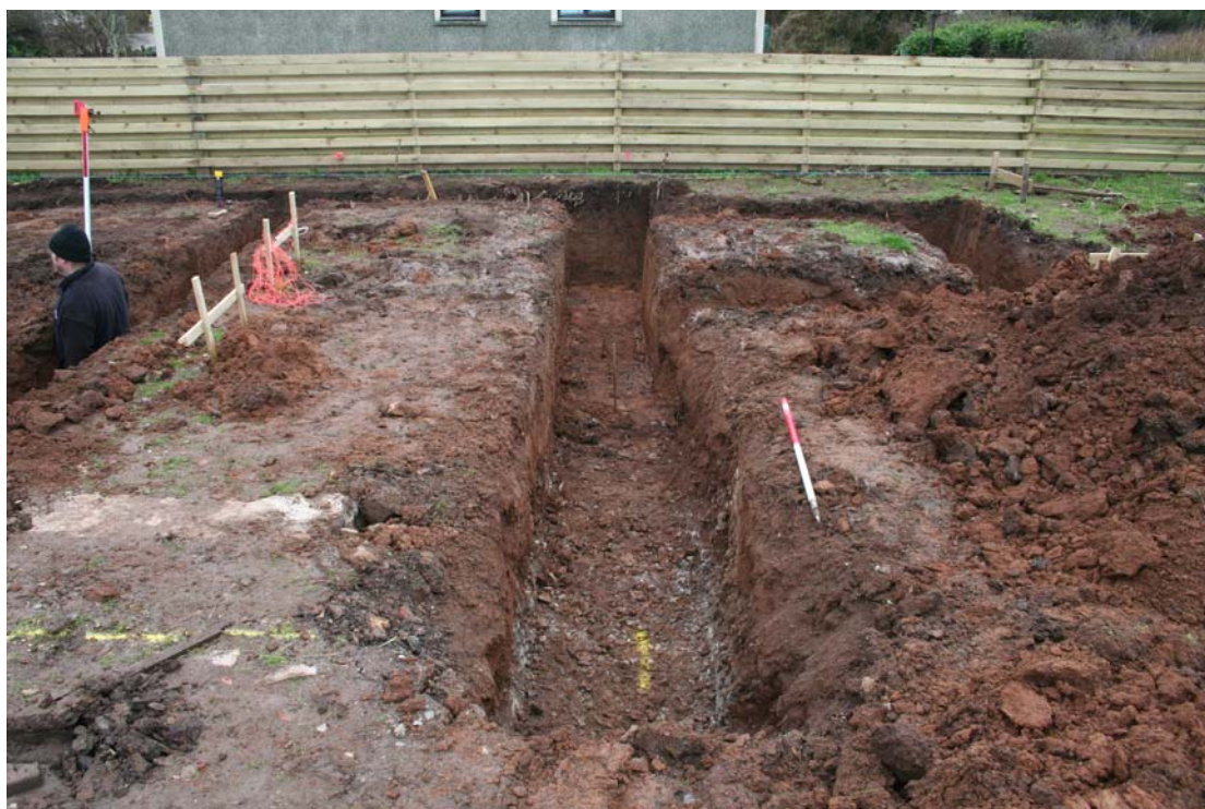
Plate 4: Post excavation shot of foundation trenches.
