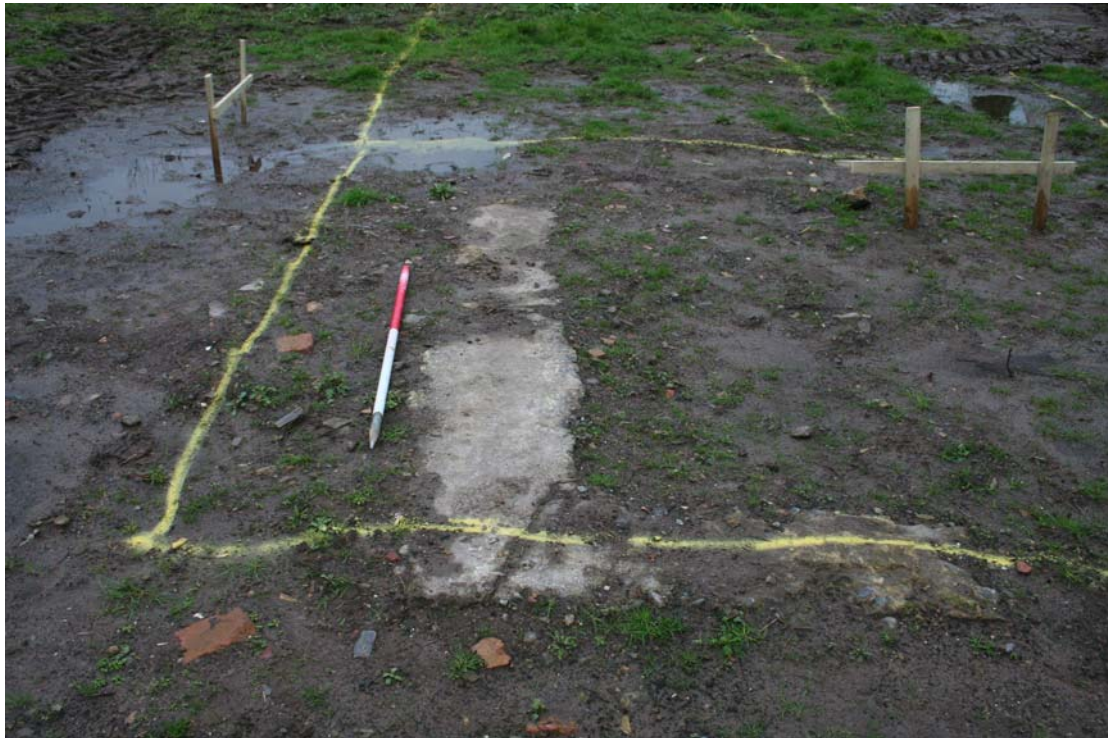
Plate 1: Surviving concrete footing associated with former cottage on site.
