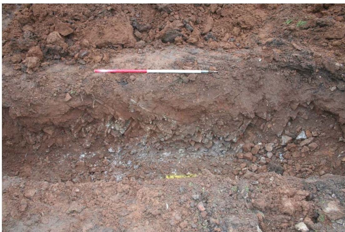
Plate 5: Shale outcropping noted in foundation trench.
