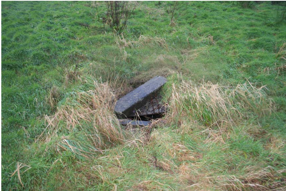
Plate 3: Damaged section of the culvert.
