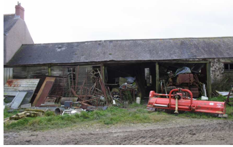
Rear of the second long farm building, with timber and corrugated iron lean-to.
