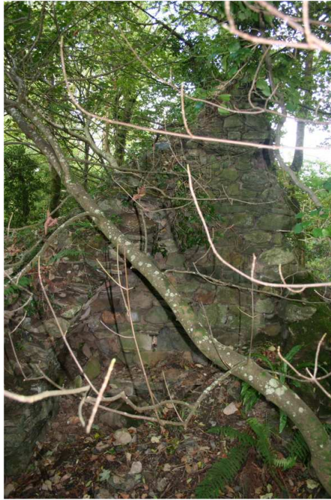
Facing north-east- the remains of a corbelled fireplace surviving inside the farmhouse.
