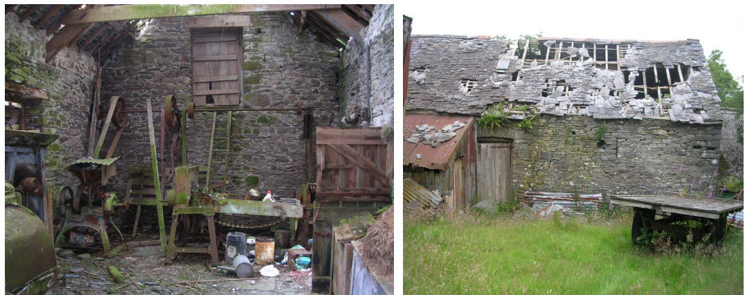
(Left), interior of the threshing barn, looking south towards access to the hay-loft with belt driven machines still in situ. (Right), rear of the threshing barn with, on the left of the picture, the engine-house for running the threshing machines.
