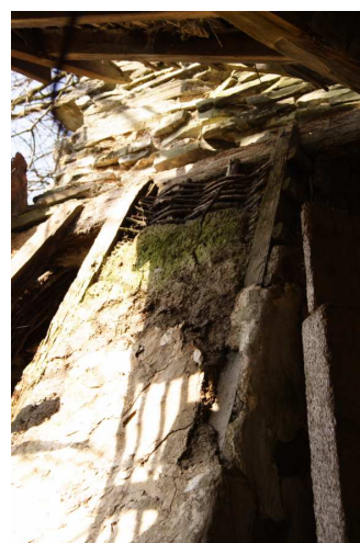
(Left) the widened gap in the southeast side wall and (left), surviving wicker-work on the chimney breast.
