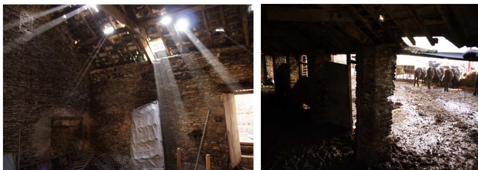
(Left) interior of the threshing barn showing gaps in the slate roof and (right) interior of the stock shed, illustrating the need for roof and masonry repairs.
