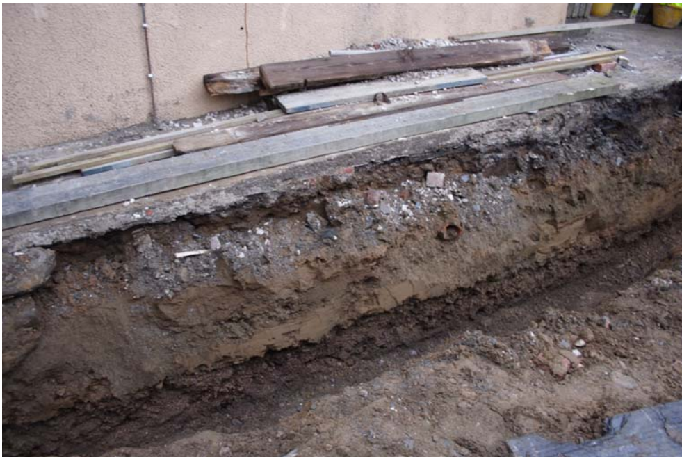
Plate 1: Foundation trench section showing natural gravel overlain by natural sand with modern construction layers at the top. View to east.
