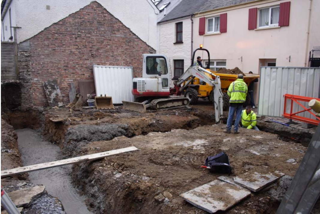
Plate 2: New foundation trenches near completion. Note the scar of roofline of the former cottage in the adjacent property.
