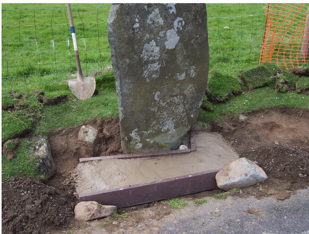
Picture 5: the concrete 'buffer' in place at the base of the stone. The square shape of the base meant that it was possible to use rigid beams of recycled plastic rather than plastic sheeting. No voids were left between the plastic and the stone's base.
