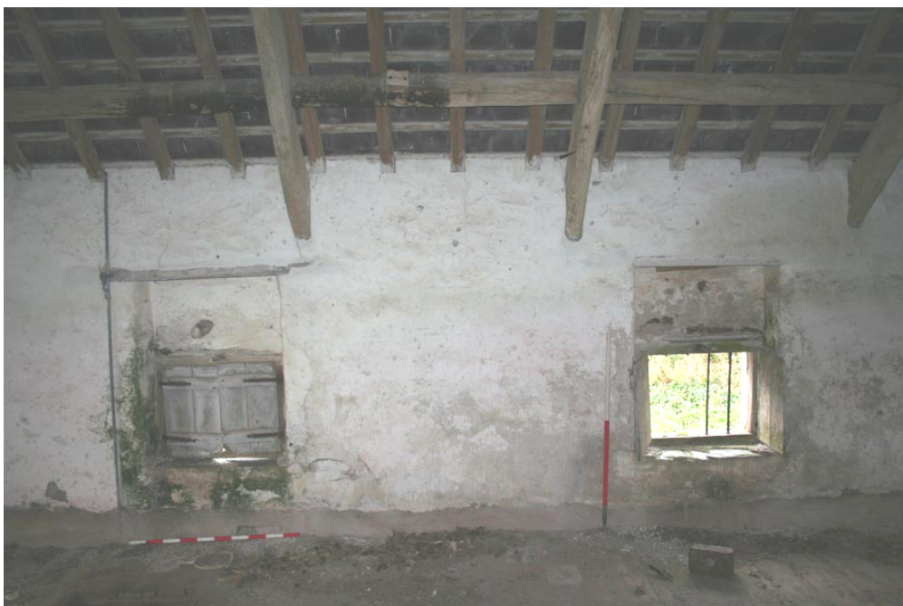
Photo 28: Detail of upper floor openings in south wall of granary
