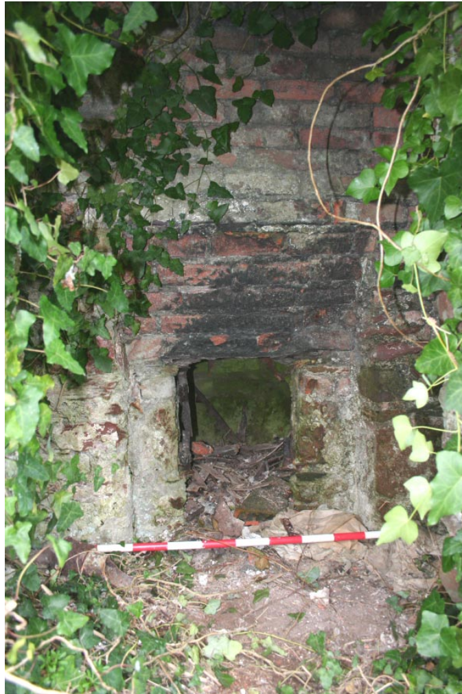
Photo 17: Stoking hole/ hearth of grain-drying oven
