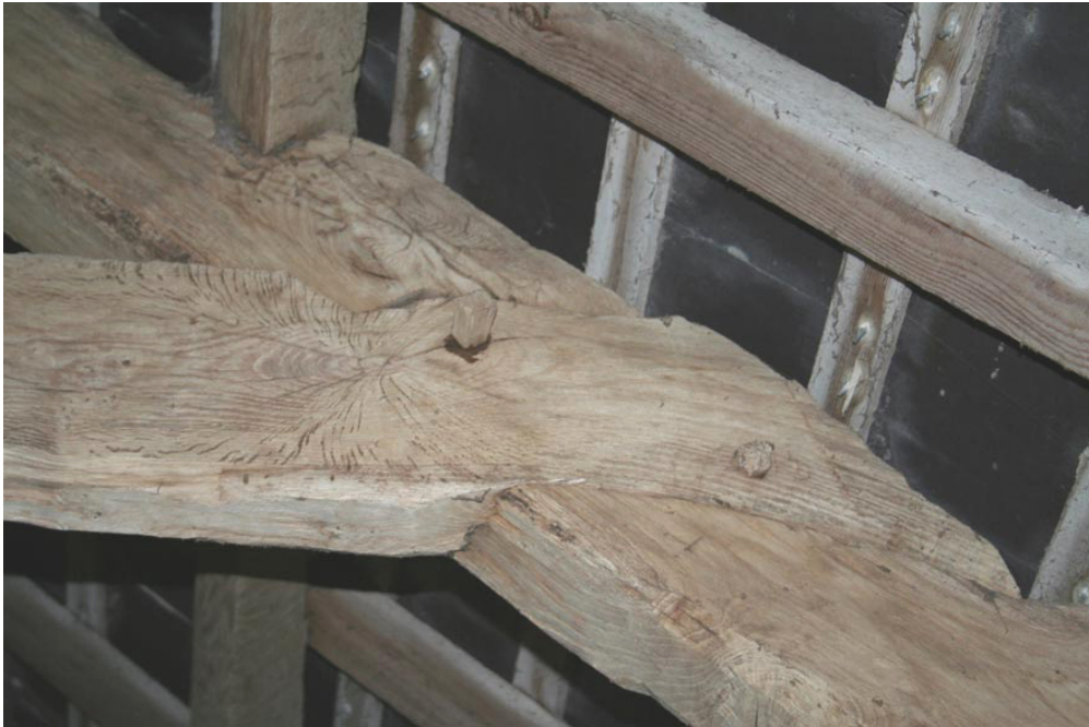
Photo 29: Detail of pegged joint in collar truss
