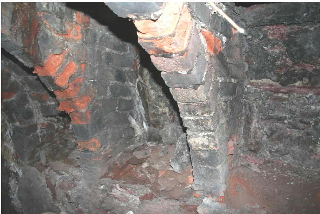
Photo 20: Brick arches supporting floor of oven (from below oven floor)
