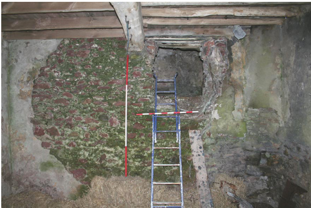
Photo 22: Damaged opening to oven interior
