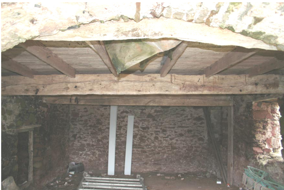
Photo 26: Beams and joists supporting floor of granary
