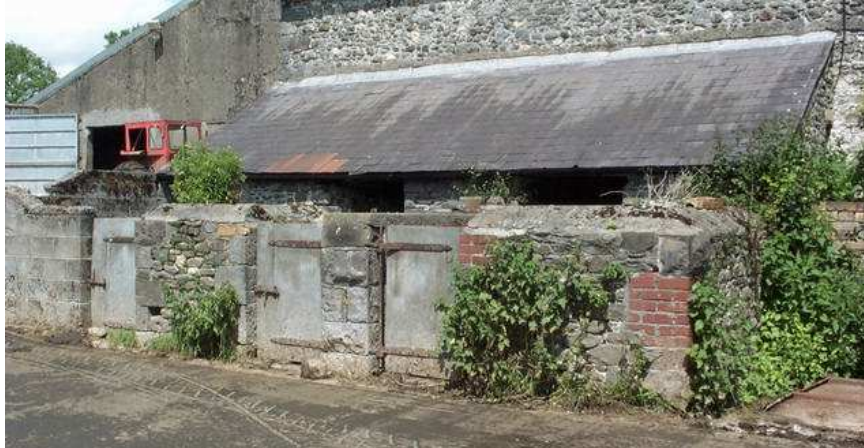
Plate 6: These pigsties at Abergwenlais Farm, Cilycwm, follow the typical arrangement of small covered pens with external yards.
