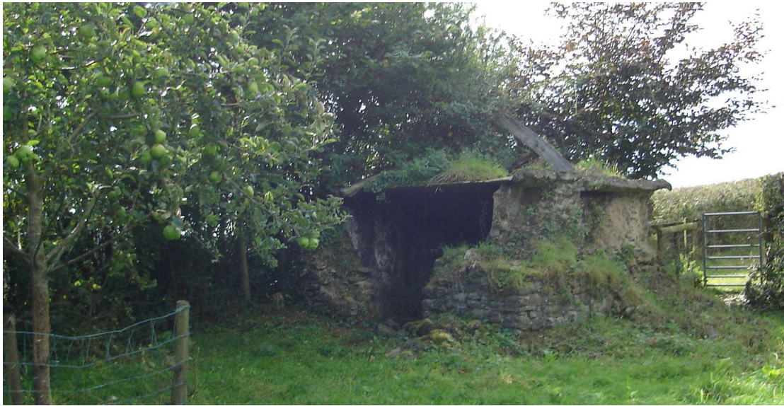
Plate 9: This small building in an orchard at Ty Pica farm, Llanegwad is constructed out of earth, built up on dwarf stone walls.
