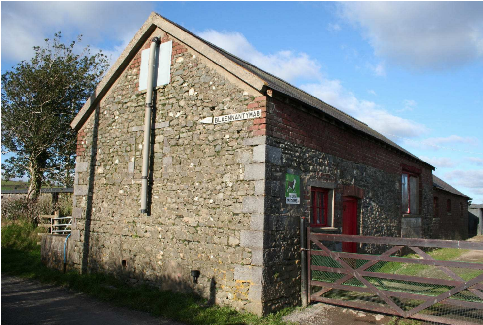
Plate 8: This modest farm building at Tir Domen, Llanegwad exhibits a hierarchy of building materials and techniques relating to the visibility of elevations.
