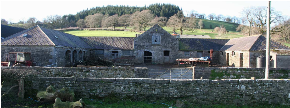
Plate 11: Cilsan, Llanegwad, this wonderful example of a small scale courtyard plan farmstead exhibits open slating, which was obviously used for decorative effect.
