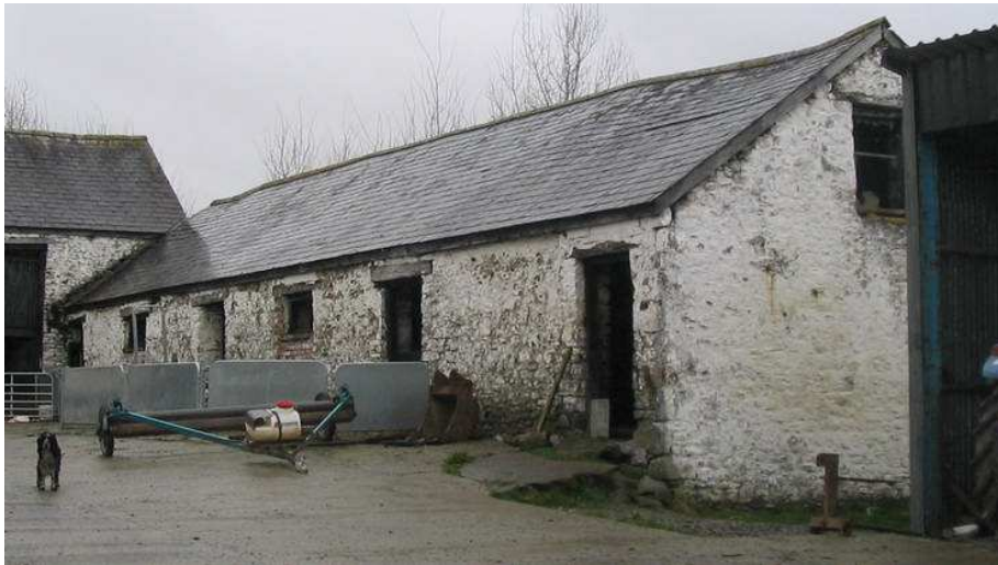
Plate 4: Gilwen, Cilycwm, cow shed, a typical arrangement of low openings with loft above.
