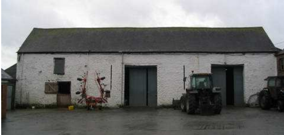
Plate 3: Pentre Meurig, Llanwrda, has a large barn with double threshing floors; typical of the Tywi floodplain
