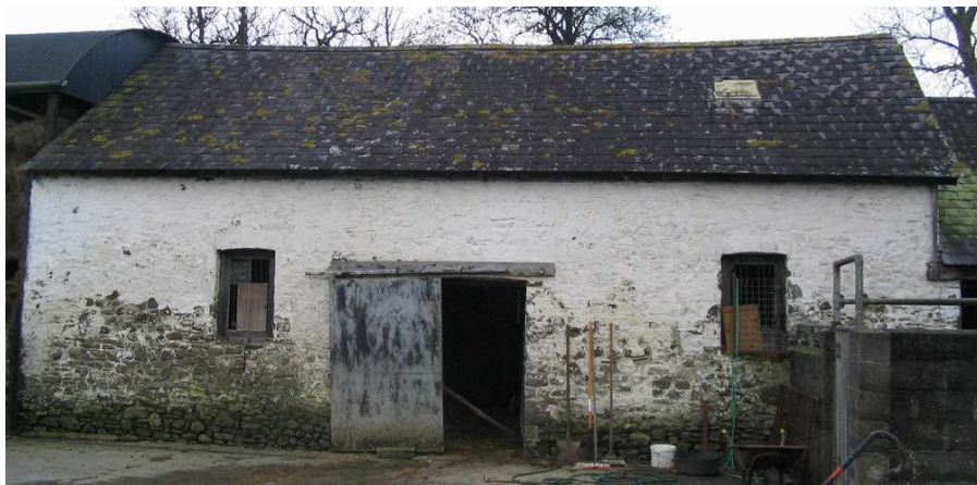
Plate 5: This stable at Glanmynys farm, Llanwrda has a higher roof line than the cow shed (to the right) and is well lit with two flanking windows.
