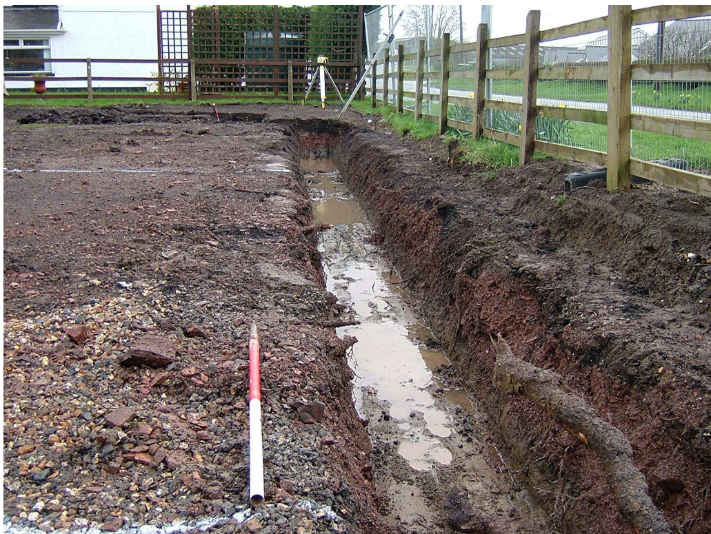
Plate 2 Line of footings dug running parallel to the Roman Road
