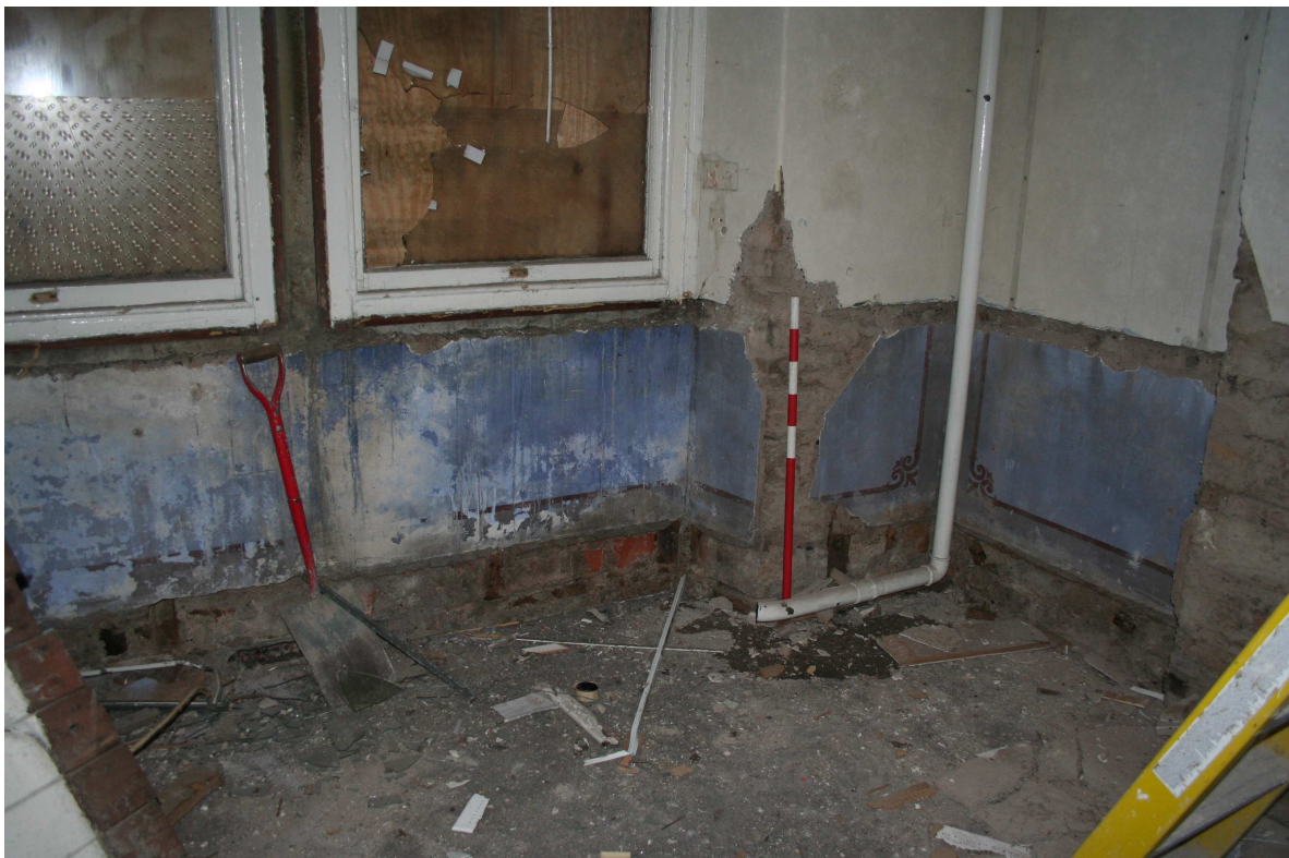
Plate 8: (1383) Interior of room west of entrance, painted plaster behind wainscot. View NE. Scale 1m
