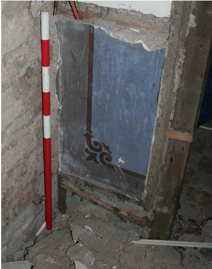
Plate 9: (1384d) Interior of room west of entrance, detail of painted plaster behind wainscot. View NE. Scale 1m
