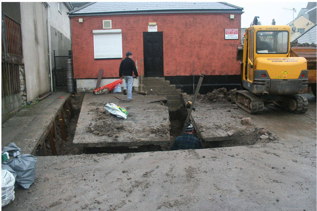
Photo. 2: Footing trenches under excavation. Eastern trench yet to be dug. View N
