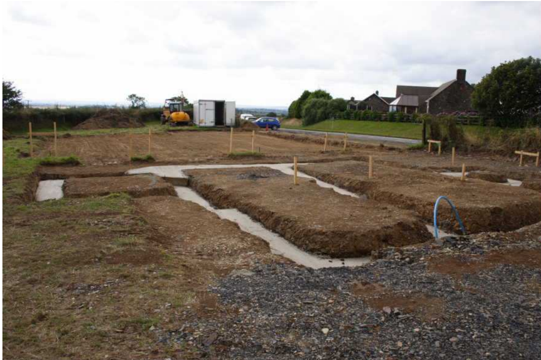
Photo.2: General view of the site area. Plot 1 footings in foreground with Plot 2 after topsoil strip, beyond, looking southwest
