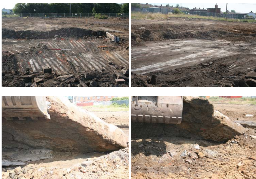
Plate 1 Concrete slab at SS5308899928, its extent, lifting and visible mesh
