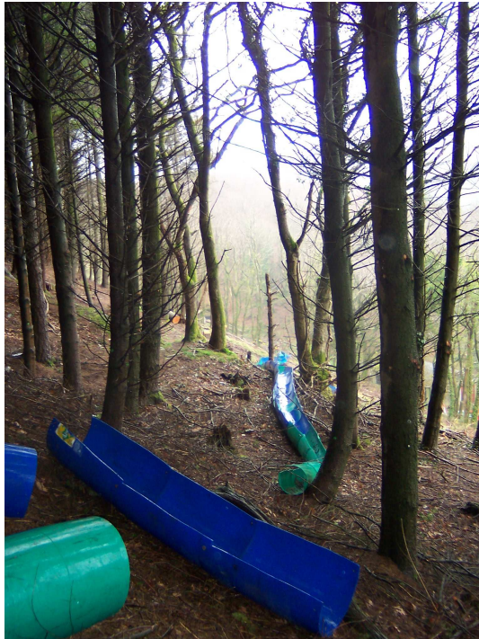
Pictures 1 and 2 (left and below) A plastic chute was constructed, and laid over the earthworks along the shallowest possible gradient.
