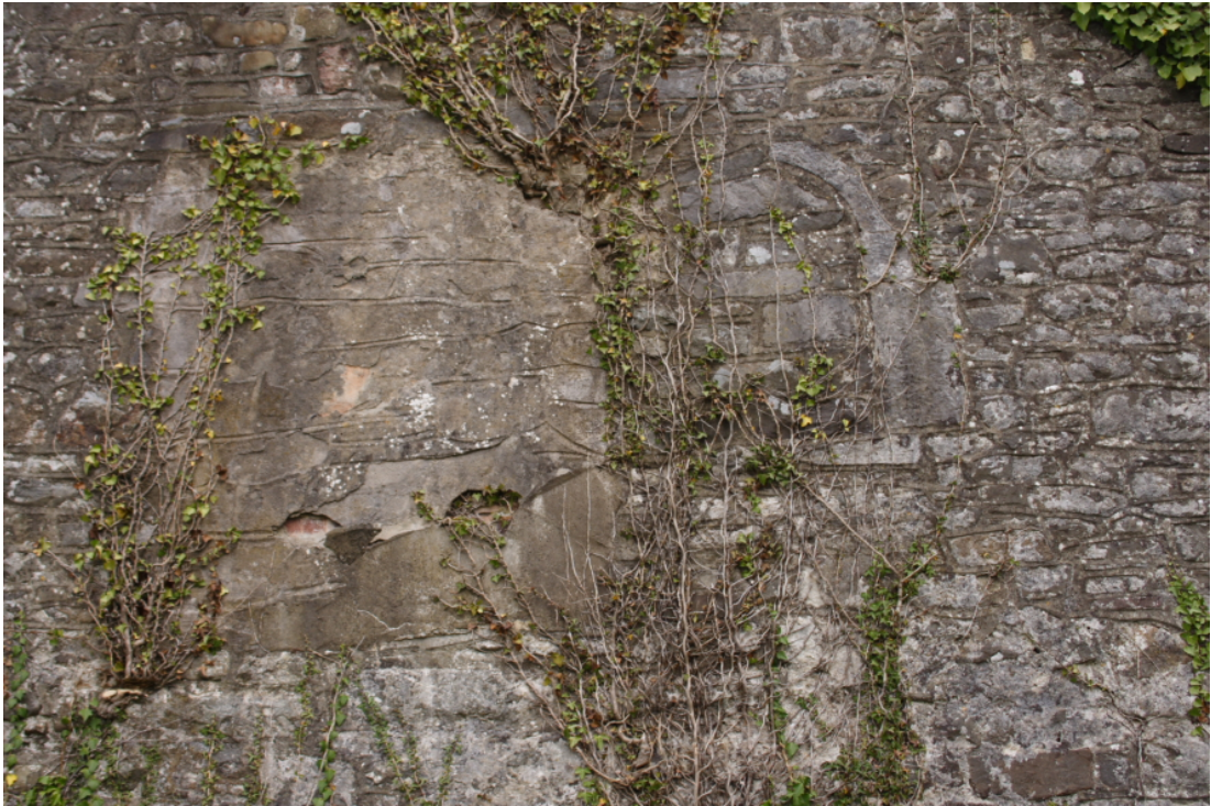
Photograph 3. Old windows in the west wall prior to restoration.
