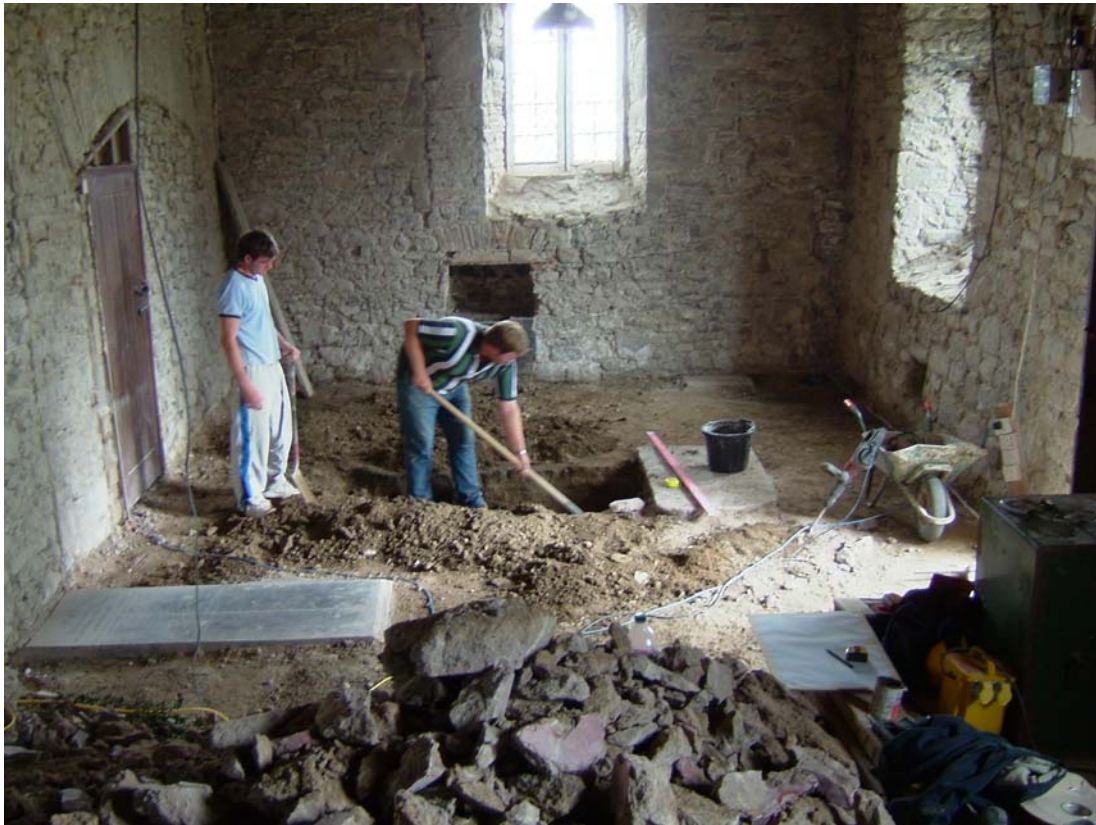
Photograph 7. Excavating the floor of the south chapel.
