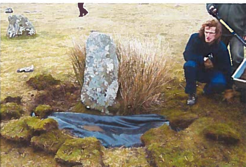
Picture 13 (above) Erosion hollow lined with Terram and waiting to be infilled. The turf cut from a nearby ditch will be used to restore the grass cover.
