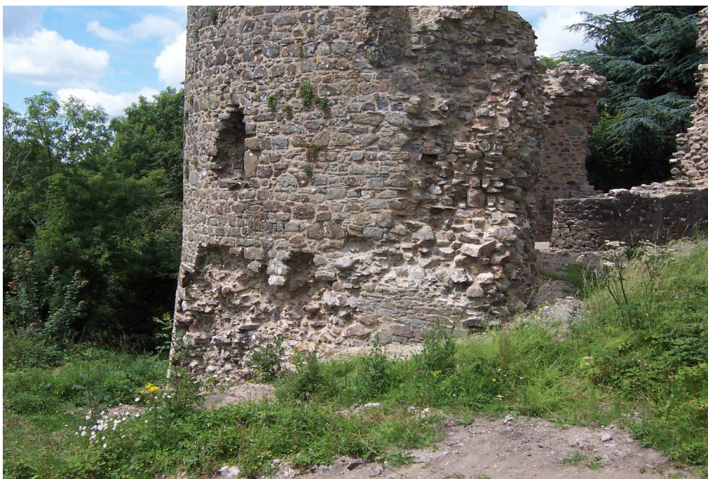
Plate 10 – The Southwest Tower from the east, after consolidation, showing facework in the area of the former ?postern
