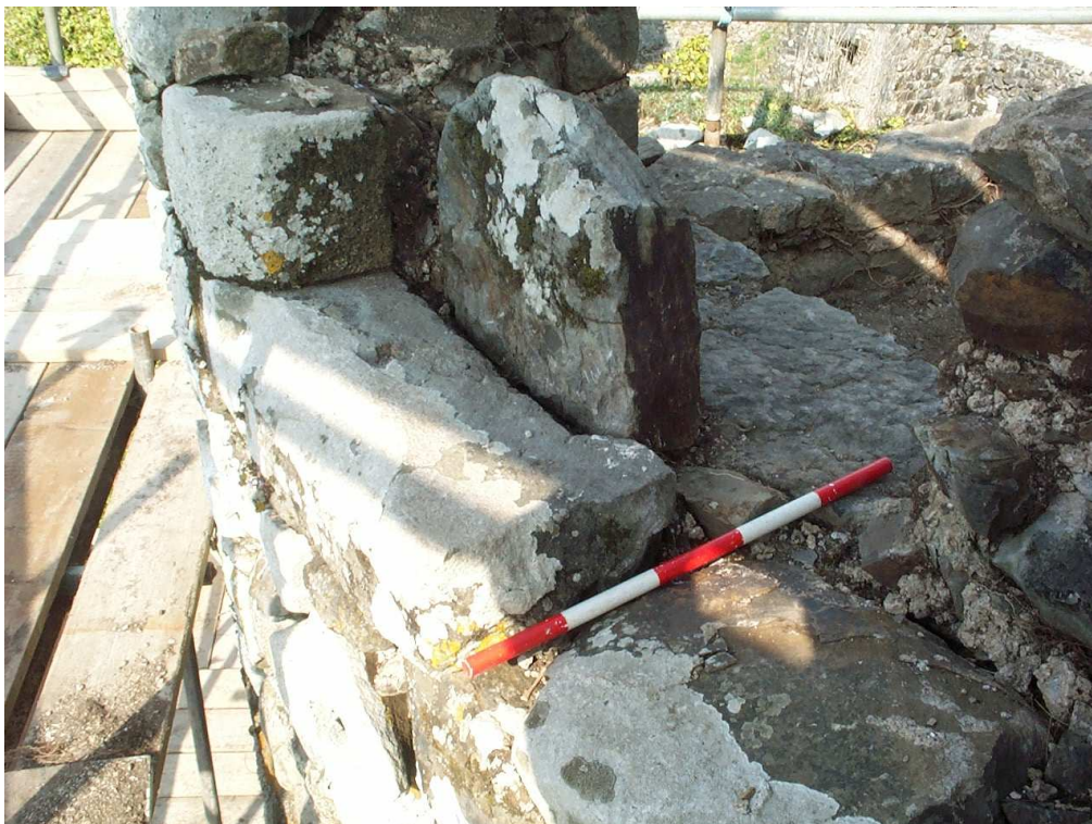
Plate 12 – Southwest Tower second floor window 3, showing the sill with in situ iron bar
