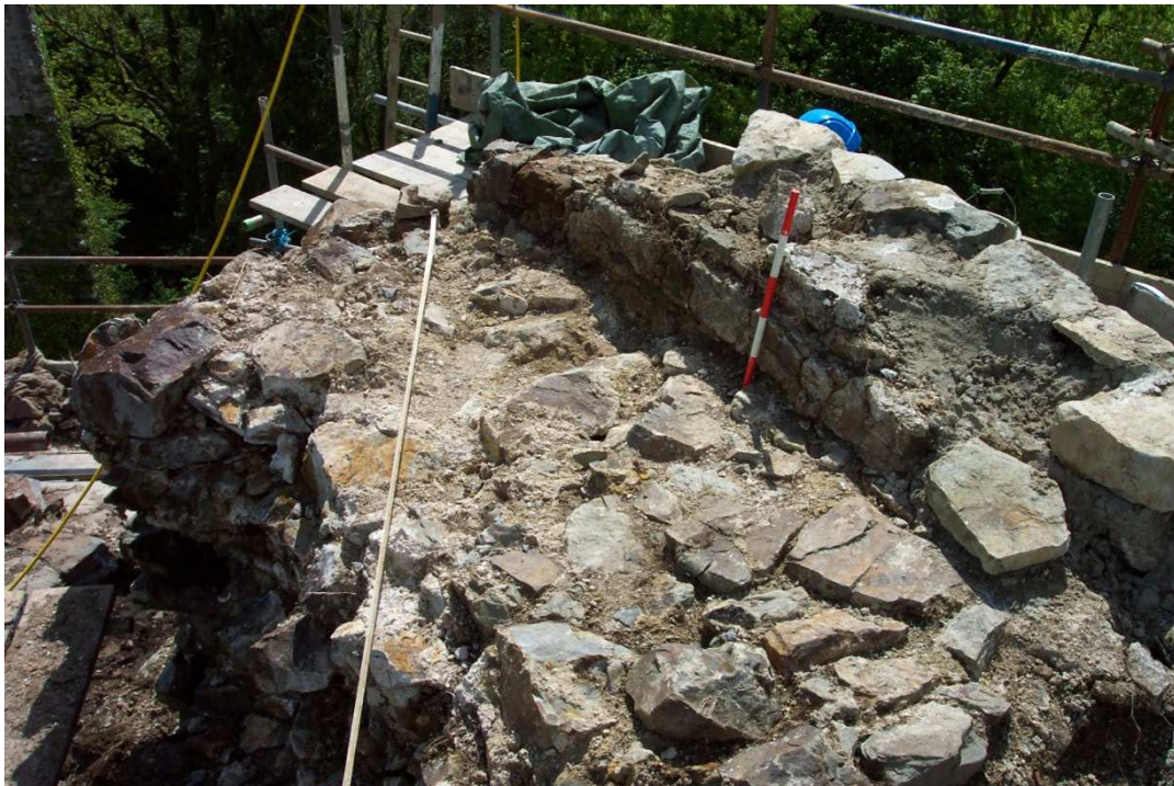
Plate 13 – The Southwest Tower: the inner face of the parapet, from the northwest, showing the offset and chase
