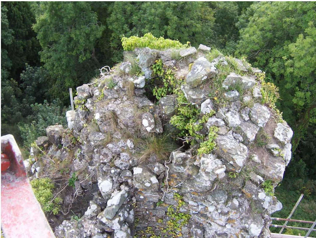
Plate 2 - The summit of the Northeast Tower prior to its truncation, from the southwest, showing window embrasure 29, and flues
