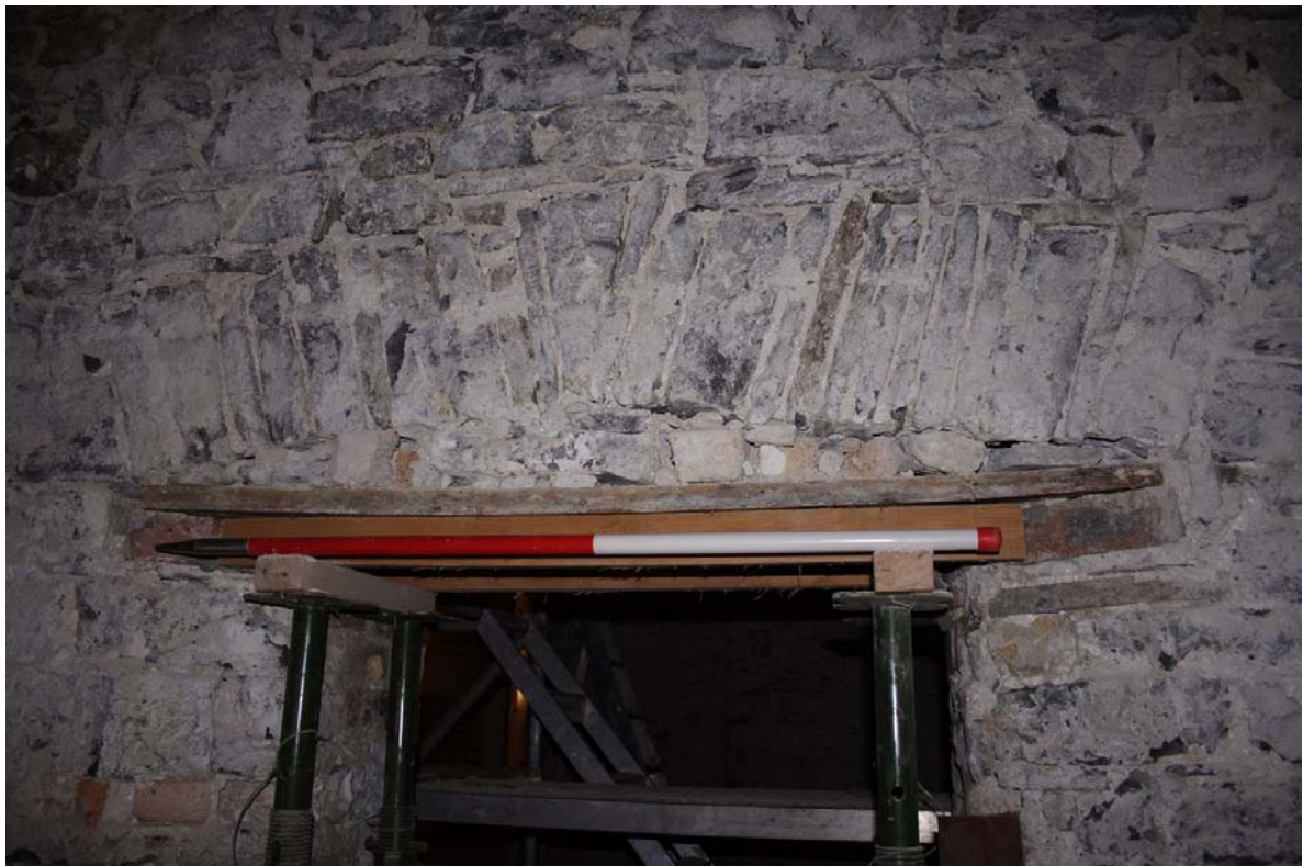
Plate 16: The stone relieving arch above the doorway to Room 4 in the east wall of Room 5.
