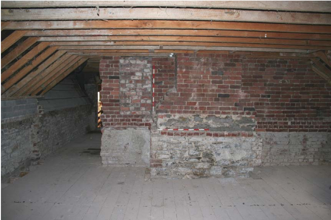
Plate 31: North wall of the attic above Room 1 showing top of chimney breast and blocked opening.
