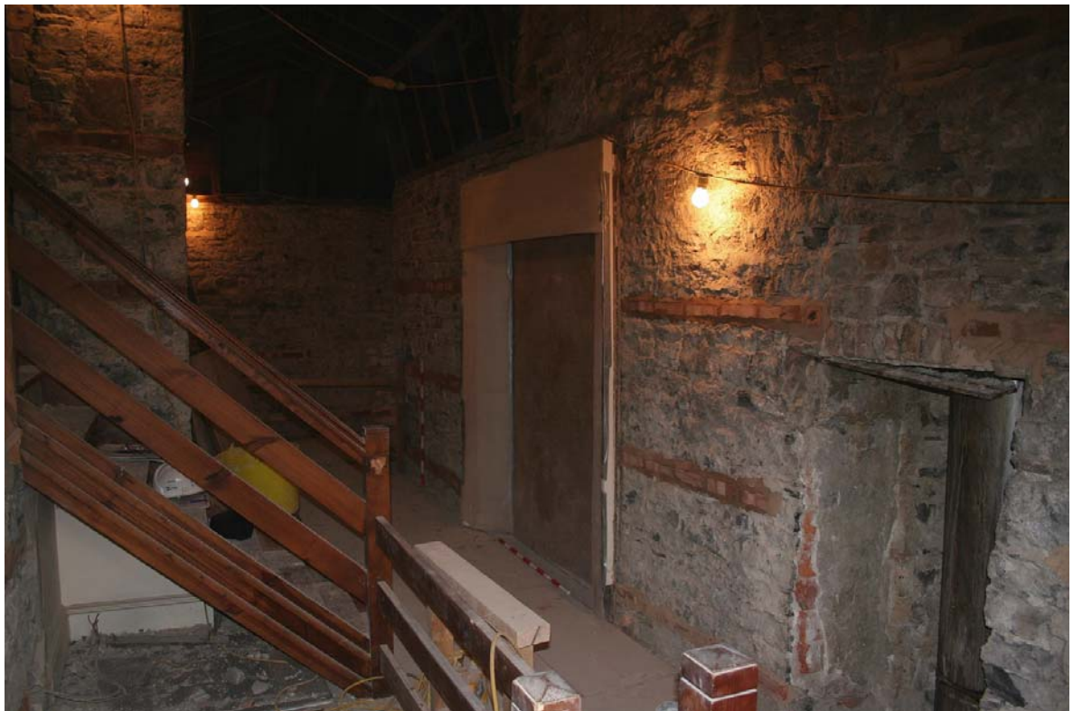
Plate 30: view south along upper level of the west wall of Room 6b showing the central fireplace and the southernmost window. Also shown are the courses of bricks inserted to replace horizontal timbers.
