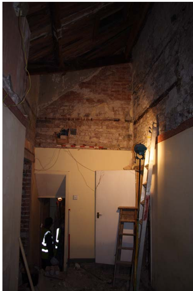
Plate 8: The north wall of Room 3, showing the old roof scar.
