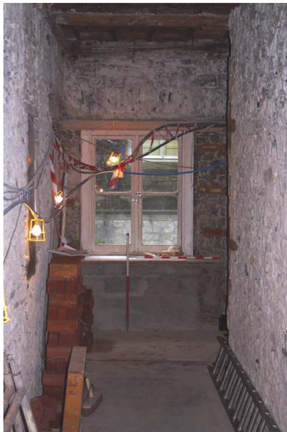
Plate 22: A former door modified into a window in the north wall of Room 6a.
