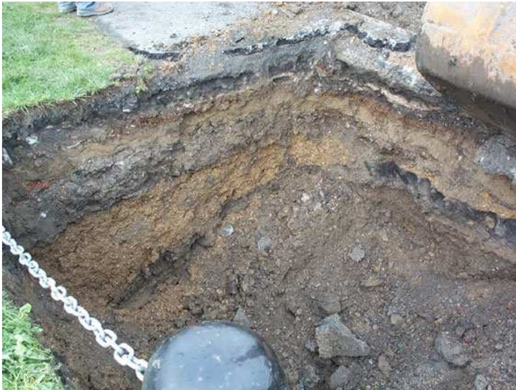
Photo 5: Backfill deposits exposed during watching brief on the new pedestrian bridge footings. Note the cobbled surface in section below the digger bucket.
