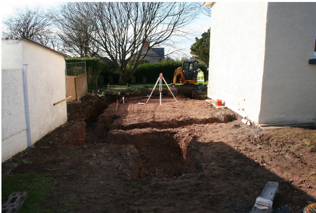
Photo 1: Footing trenches almost complete. View W
