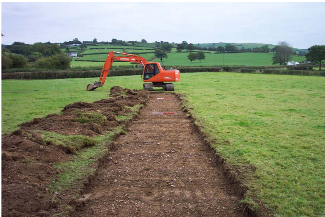
Plate 1: The centre line of the new paddock area following the removal of approximately 10cm of topsoil. The supposed Roman road line runs in front of the hedge in the background.
