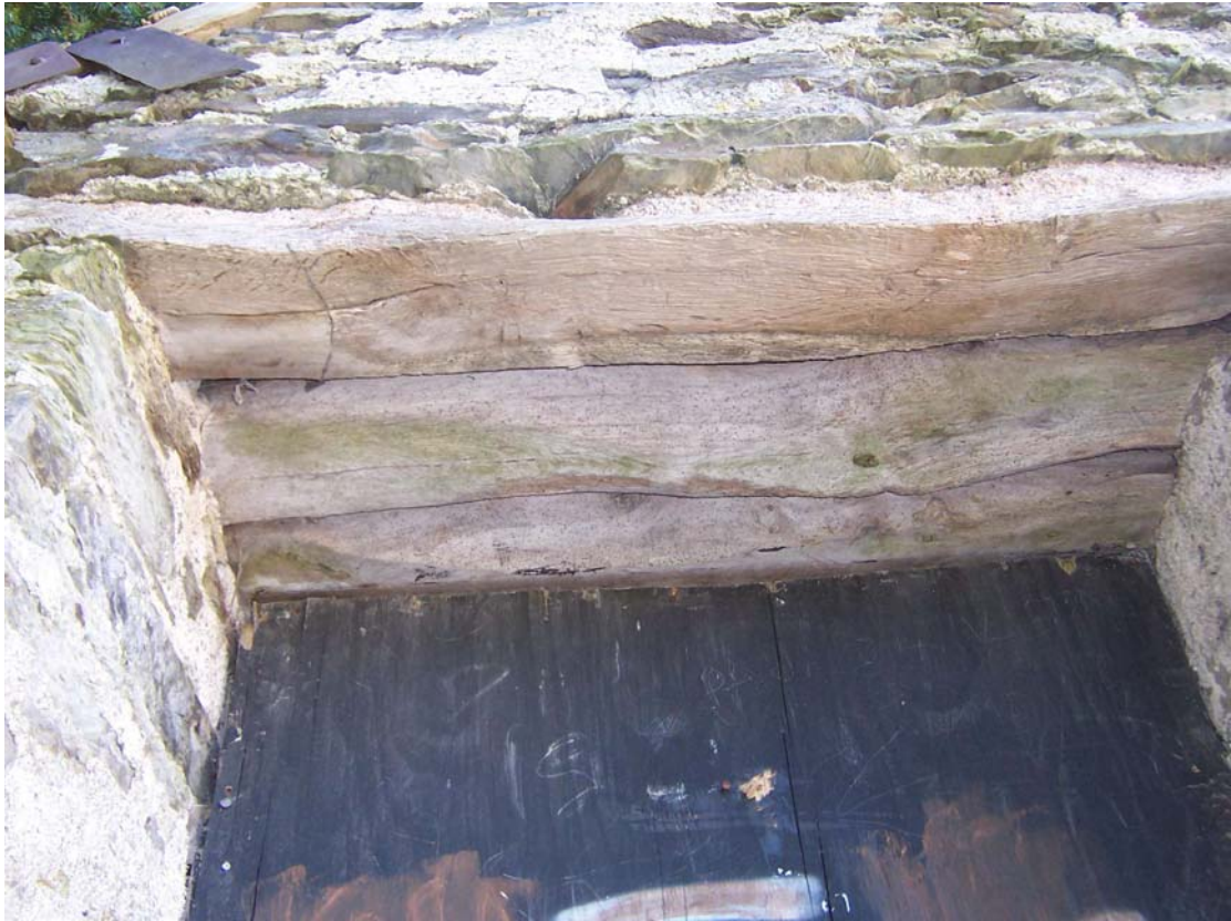
Photo3: Lintel above doorway to loft in northern gable end
