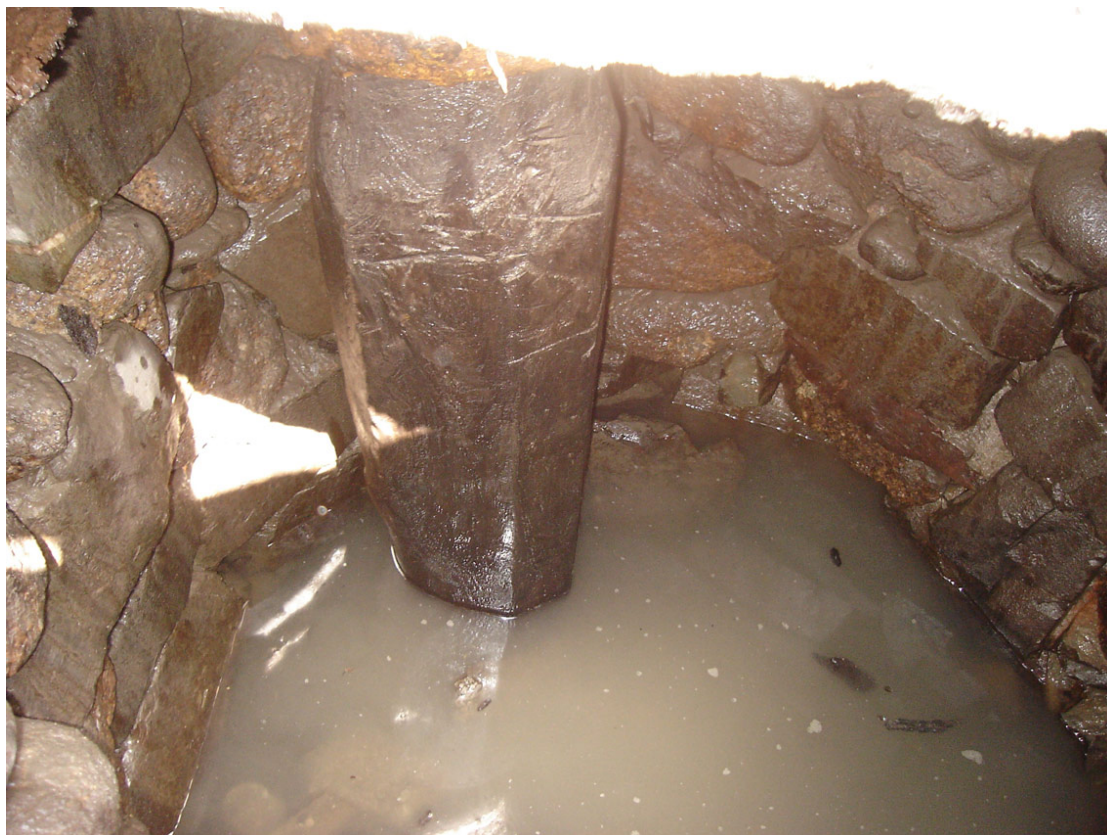
Photo 4: Hollowed timber pumping column within well structure
