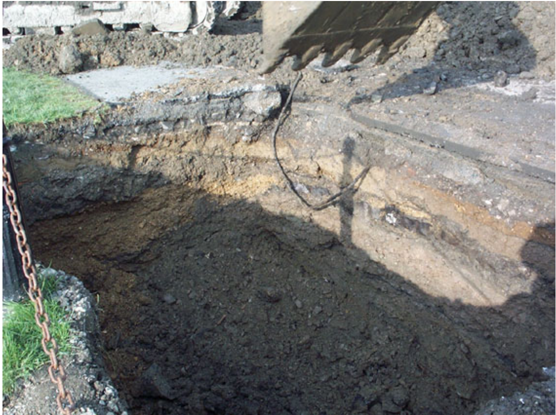
Photo 1: Make-up and backfill deposits revealed during preparation of bridge footings
