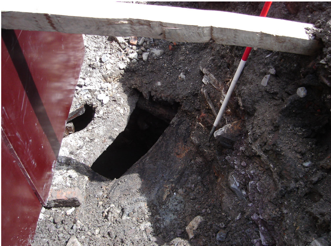
Photo 2: Scrap wood capping the well revealed during preparation of bridge footings
