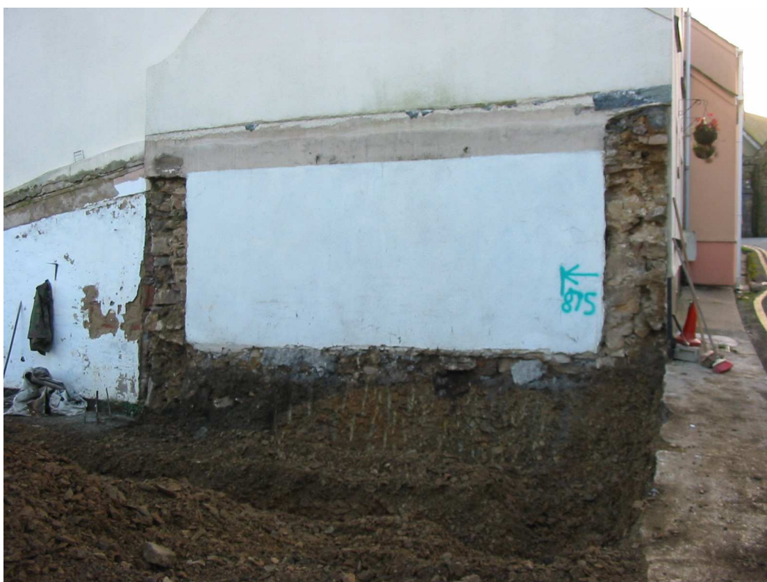
Photo 2: Cut with dark fill below gable end footing. View South West
