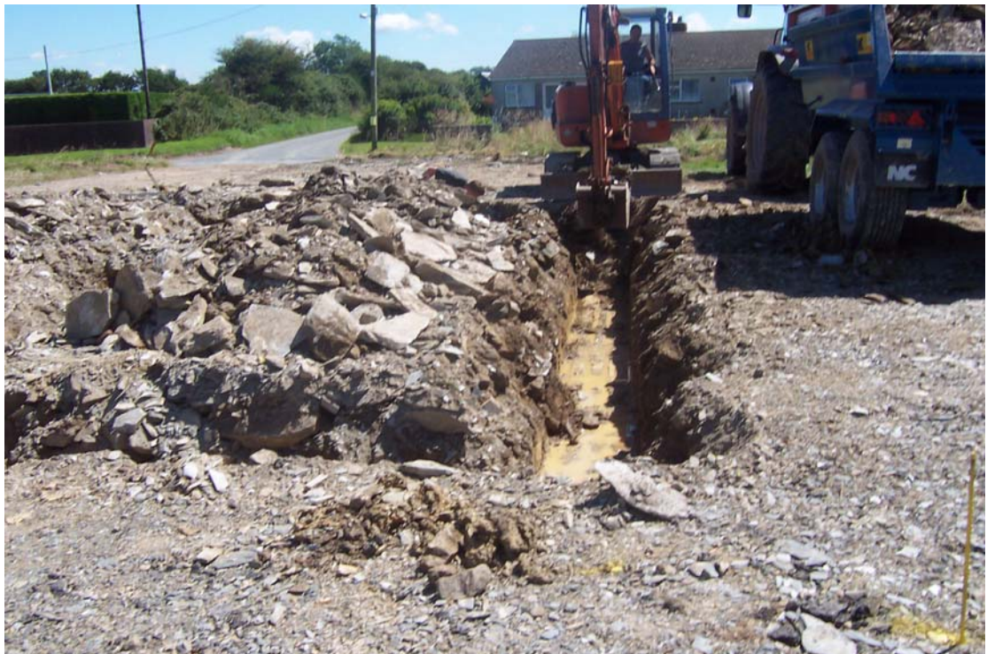
Photo 2: Southern foundation trench, hard-standing makeup on spoil-tip
