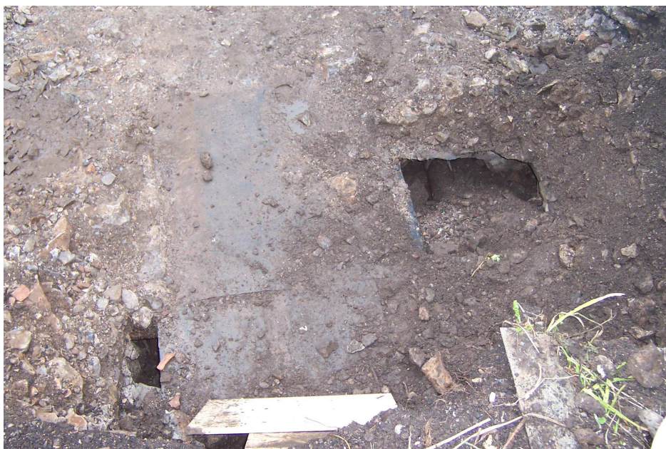
Plate 3: slate covered drain.
