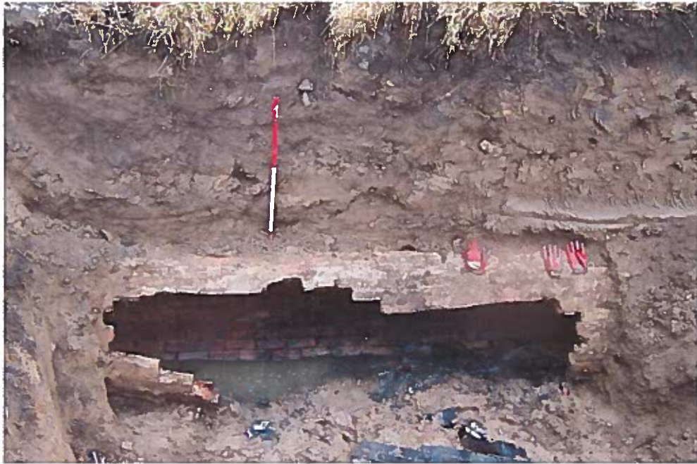
Plate 2: The collapsed section of the culvert and overlying stratigraphy.
