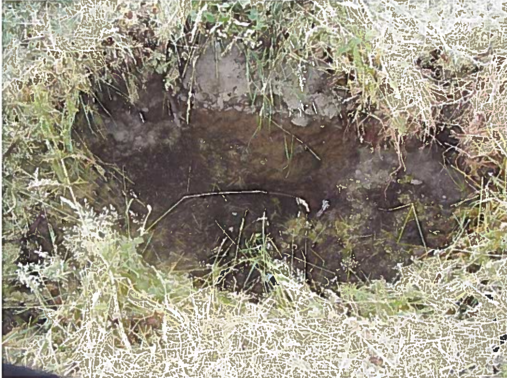
Plate 1: The hole caused by the initial collapse showing the topsoil and subsoil.
