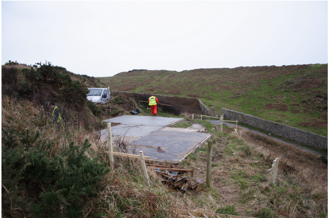
Photo. 1: Concrete raft of earlier building. View SW
