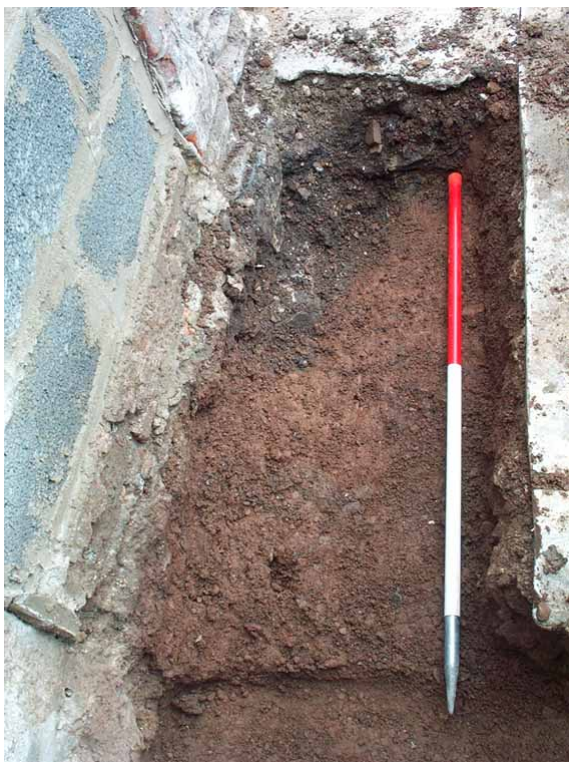
Photo 3: (lack of) Wall footings in southwest corner of original building, looking north
