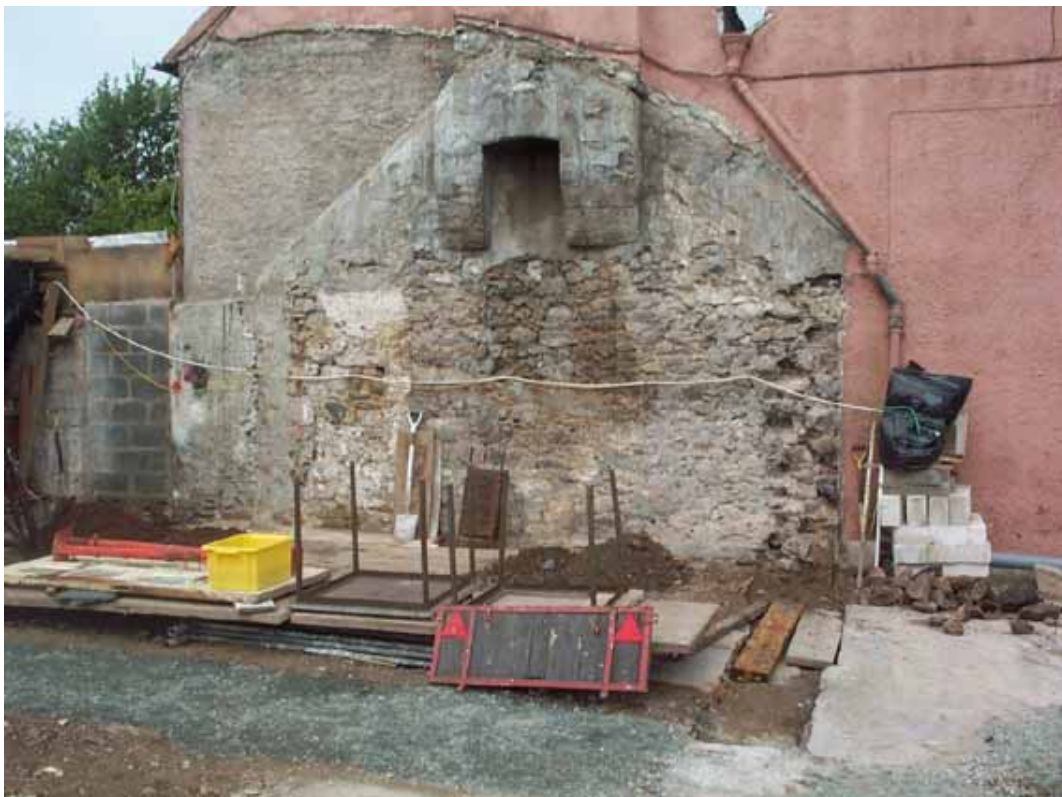
Photo 2: End wall of the Old Bake House showing wall scars and footings, looking west
