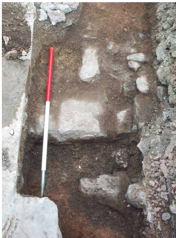
Photo 4: Footings to the southern wall of the original building, looking north
