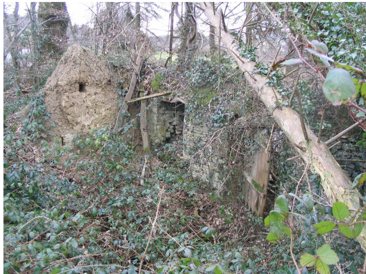
The cottage incorporates both stone and clay-walls in its design.
