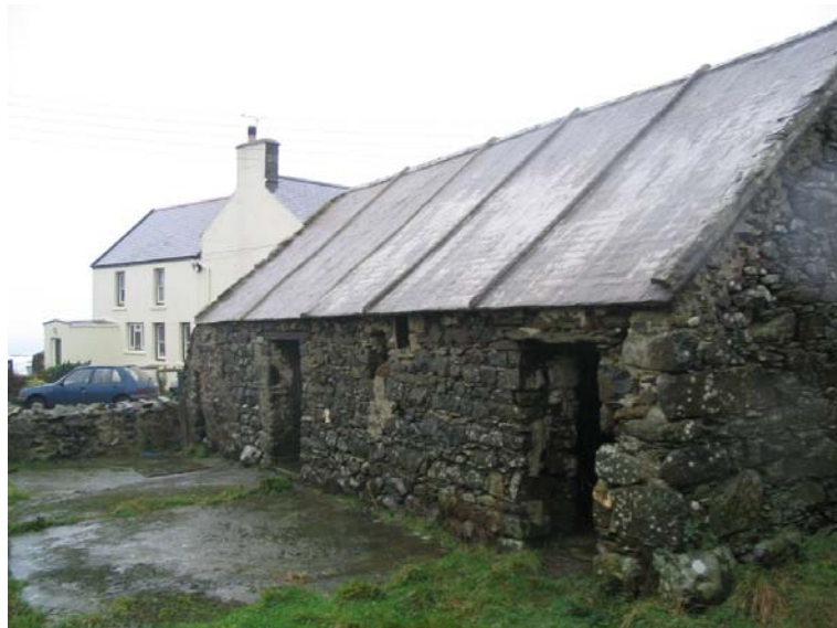
Grouted slate roofs survive in part at Pwll Caerog.
