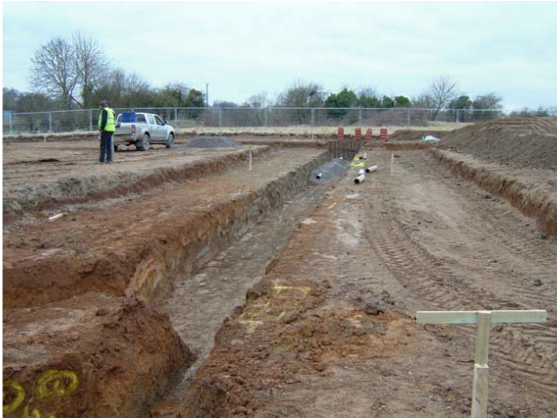
Photo 3: Excavation for drains.
