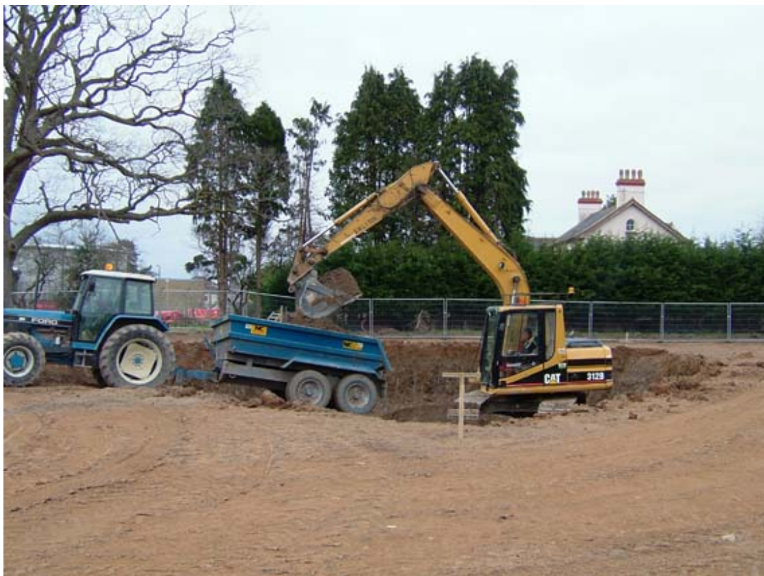
Photo 4: Excavation of the balancing pond.
