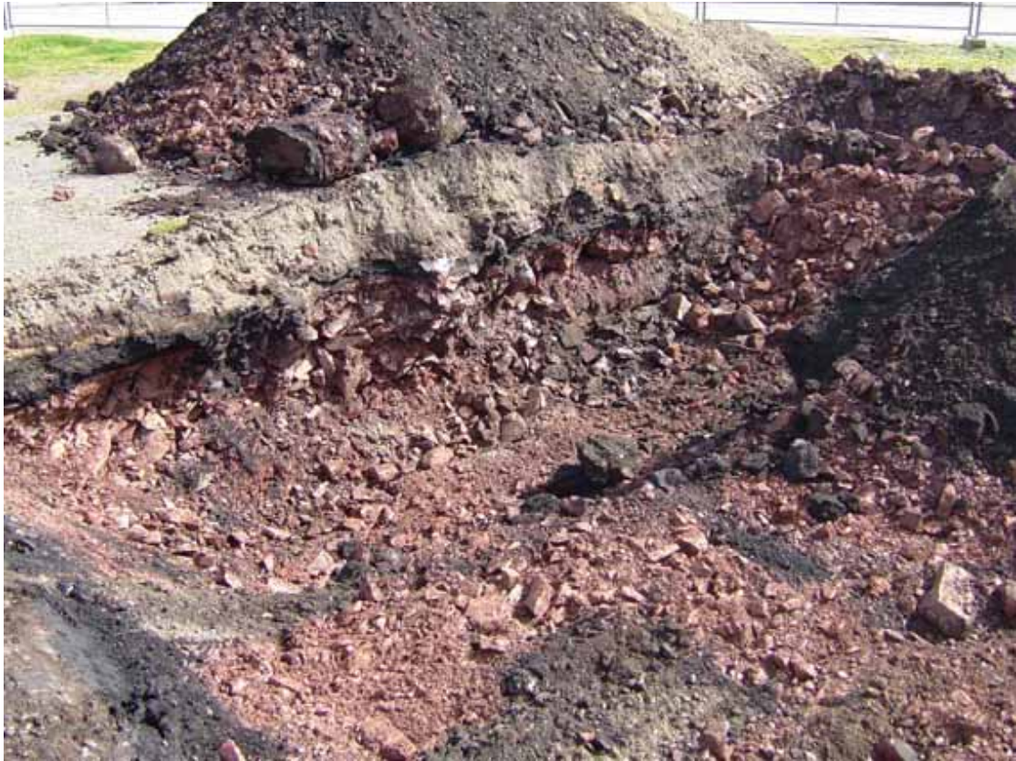
Photo 1: Stone rubble quay construction material overlain by demolition debris
