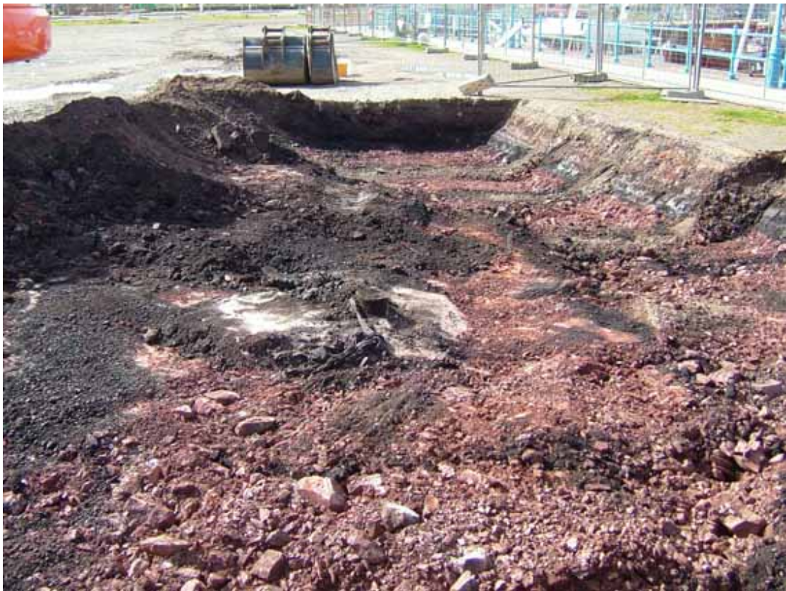
Photo 2: Concrete setting for demolished steel frame building
