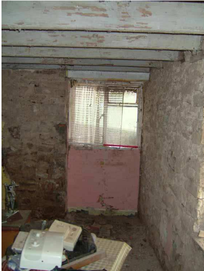
Photo 9: Doorway in north wall of room C converted to window
