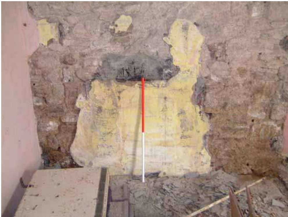
Photo 4: Blocked fireplace on north wall of room C
