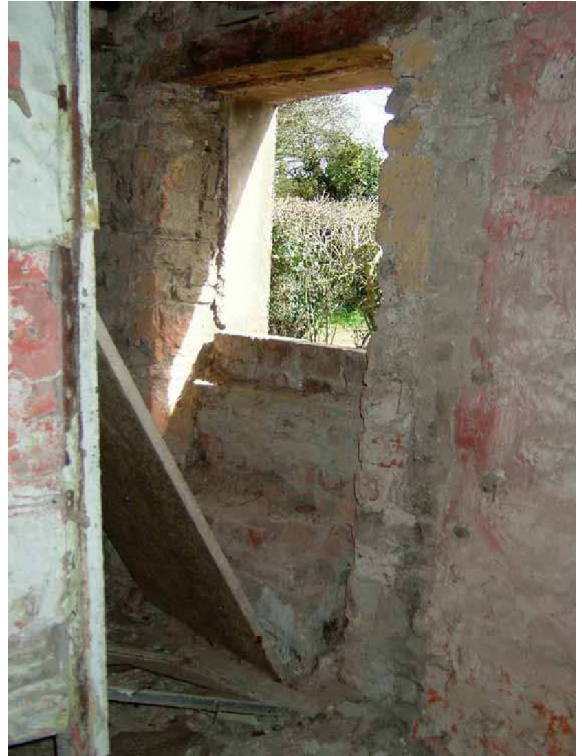
Photo 10: Doorway in east wall of room A, converted to window
