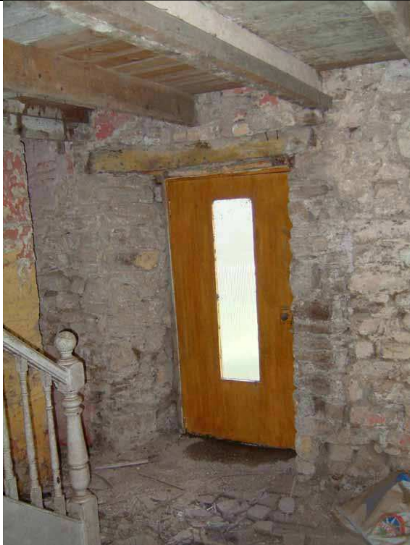
Photo 11: Doorway in west wall of room A. Note blocking on right side of doorway
