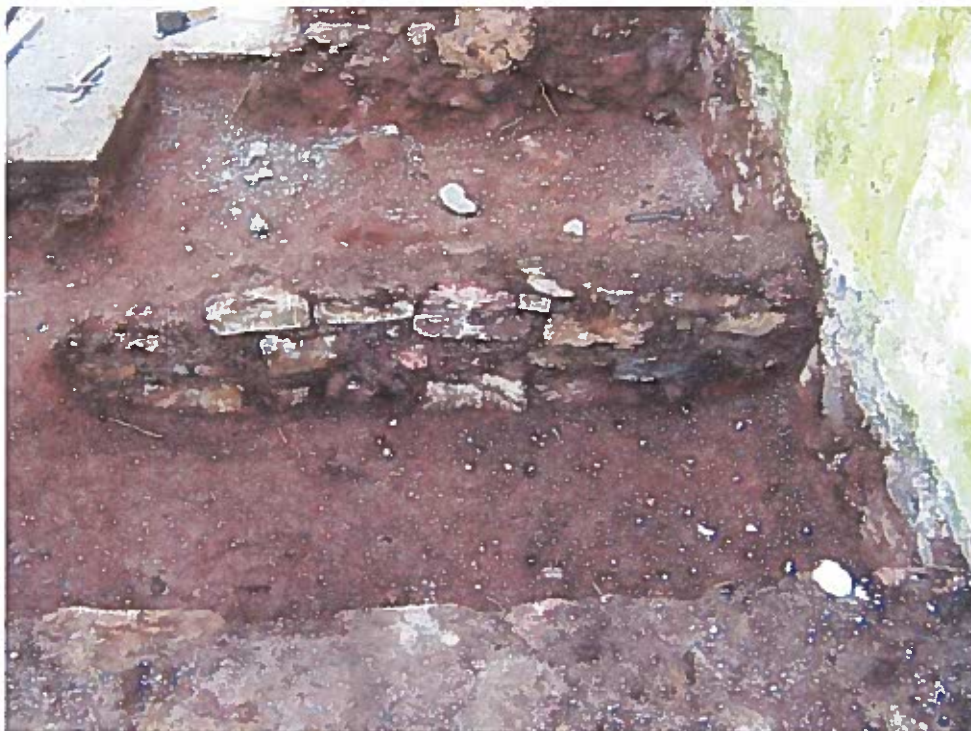
Figure 3 (below): Dwarf wall at the east end of the nave. These walls are roughly built, and butt up against the exterior walls of the church. The gaps between them were filled with modern debris from the removal of the roof and from the building standing empty. The walls are not finished neatly, but appear to have robbed out where the aisle passes through (left of picture).
