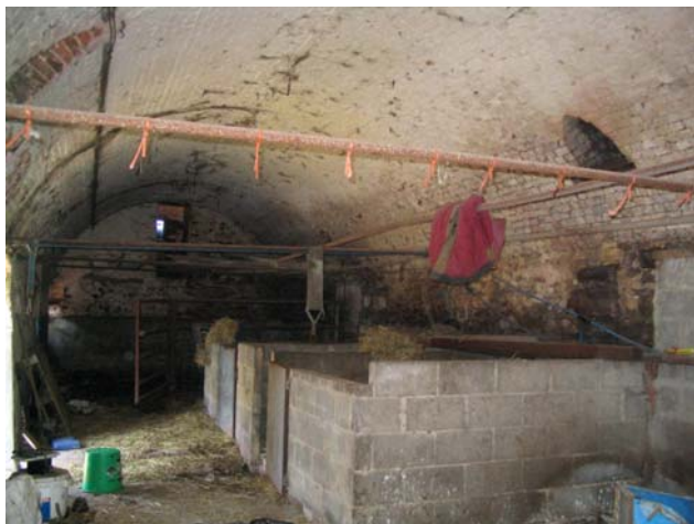
Internal shot of cowhouse in the centre of the main range of the combination farm building, showing the unusual brick vaulted ceiling.
