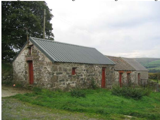
SE facing shot of the southern barn range, also showing the varying roofing materials. Slate with corrugated iron patching remains on the central barn, although in a deteriorating state.
