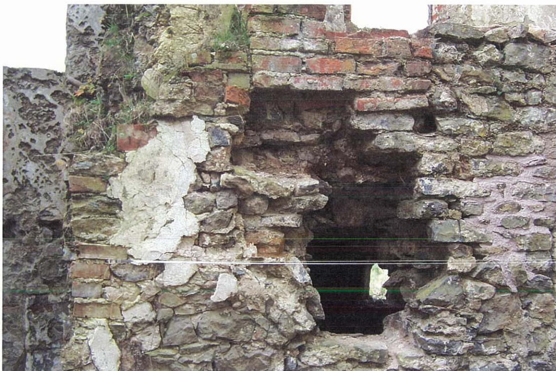
Photo 5: Detail of masonry in exterior face of undercroft wall in the vicinity of the 'window' opening
