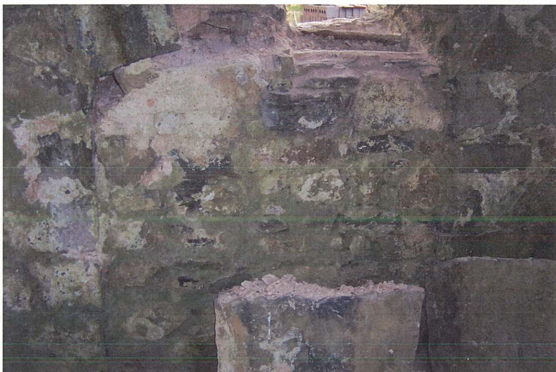
Photo 1: Blocked archway in interior face of undercroft wall
