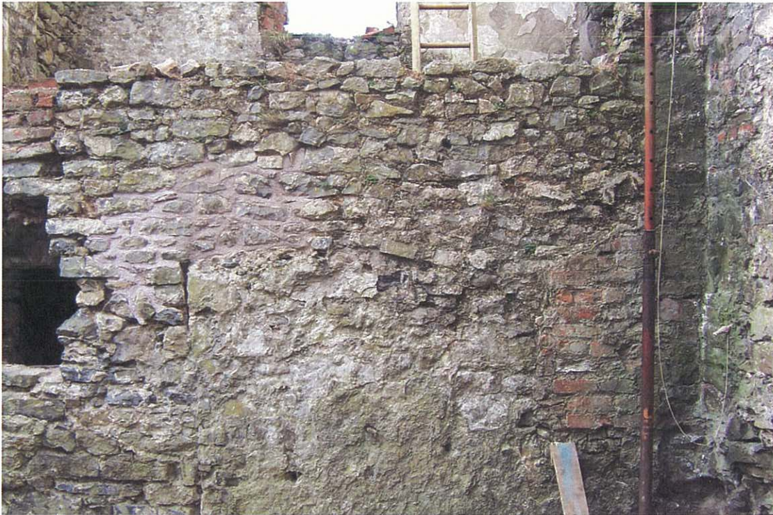
Photo 4: Shot of east facing elevation of undercroft wall showing various masonry builds
