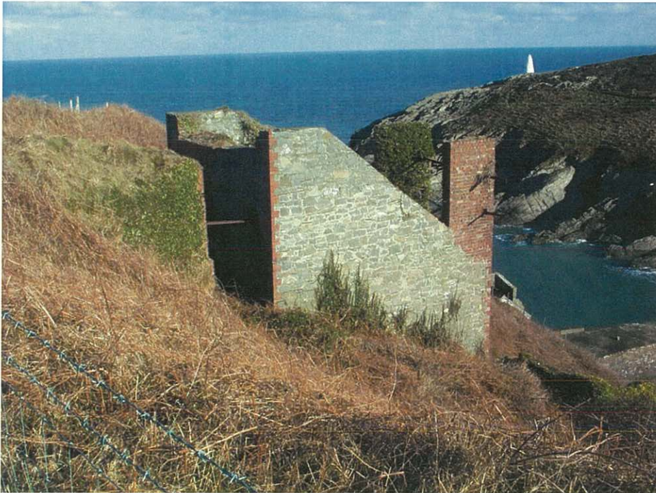
Plate 10: The feed platform for hoppers 13-15.
