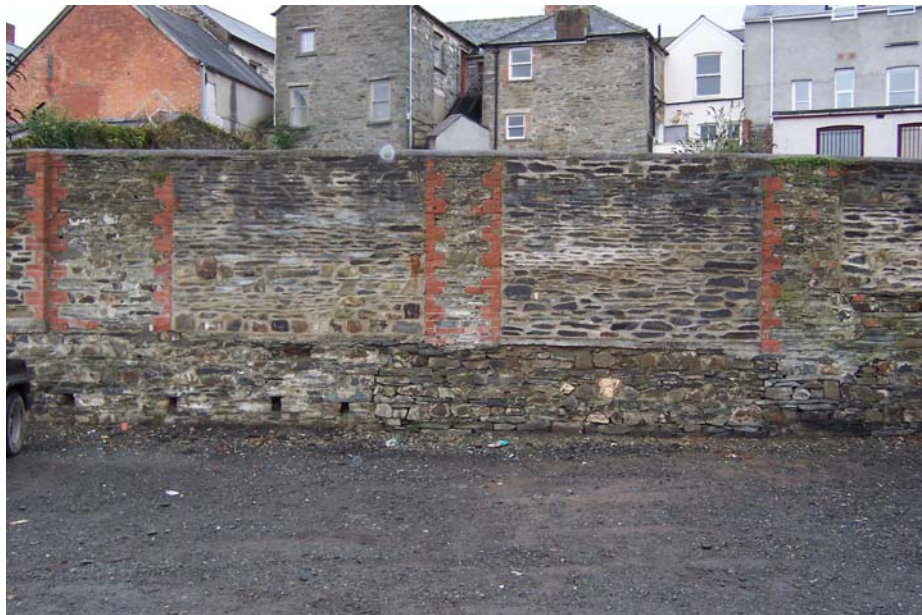
Plate 4: The west wall of the Black Lion Inn car park showing the blocked openings, probably from a row of garages demolished in the 1970s. Chancery Lane lies behind the wall and the concrete layer at the bottom of the brick quoins marks the current street level.
