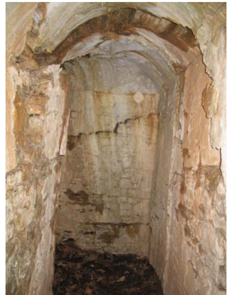
The entrance passage, cracked and contorted by tree roots
