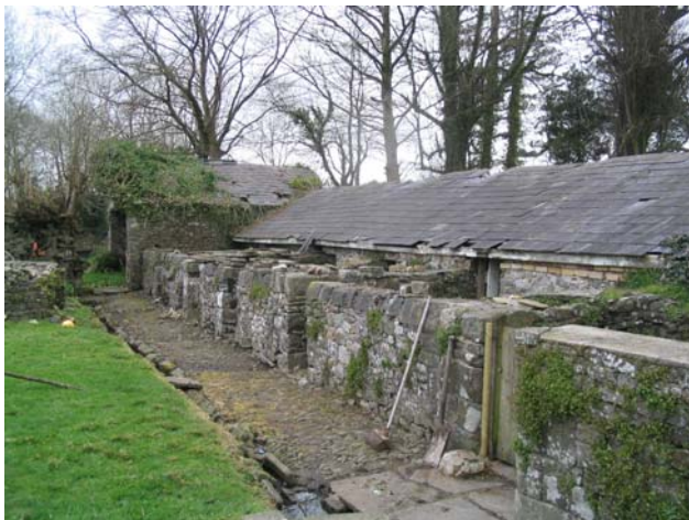
The long range of pigsties with a pitched stone apron and drain to the front.
