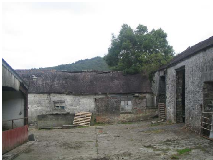
The inner face of the northern barn range, showing the dilapidated state of the roof. The large threshing barn doorways of the eastern range are visible to the right.
