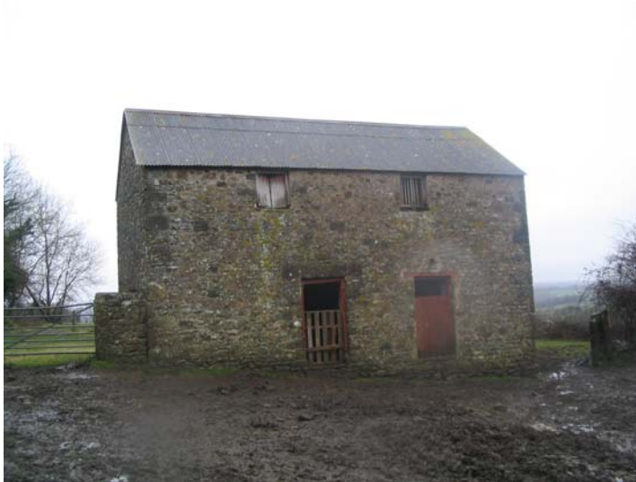
Southeast elevation of two-storey building described above, showing lowered ground surface and exposed foundations
