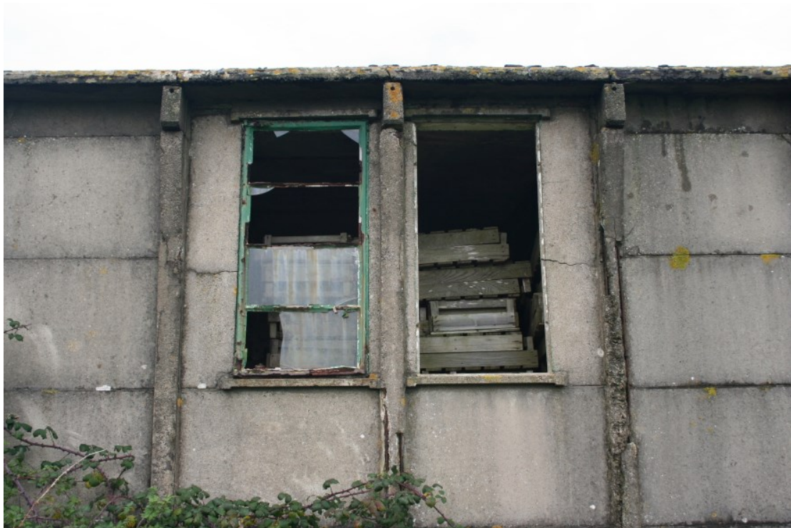
Plate 7 – Exterior detail of casement windows in the eastern elevation of the Wireless Telegraph Hut (PRN 28642)
