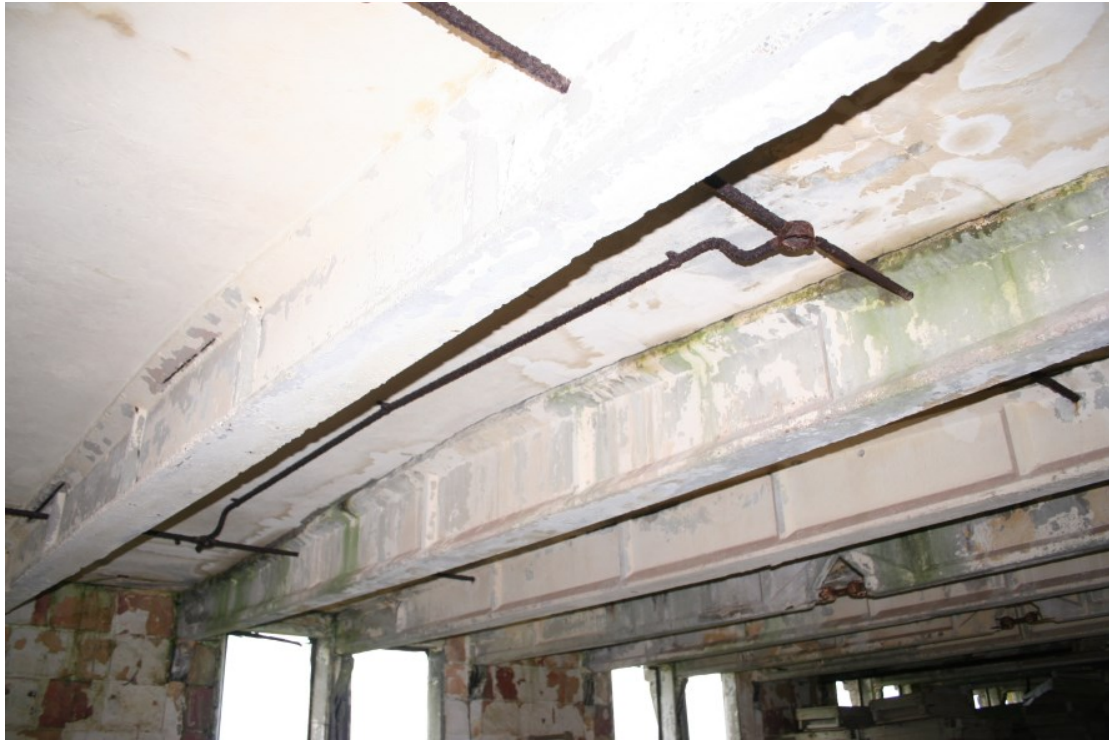
Plate 3 – Interior of Wireless Telegraph Hut (PRN 28642), showing electrical conduits, also note steel tensioning in two of the concrete roof trusses.
