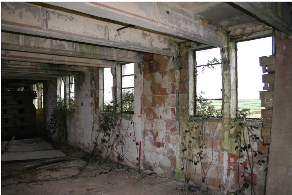
Plate 2 - Interior of Wireless Telegraph Hut (PRN 28642) showing interior clay blockwork and concrete roof trusses.
