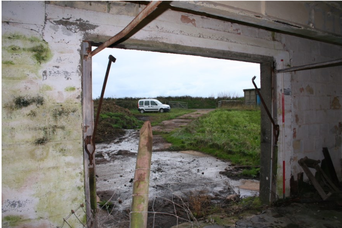
Plate 5 – large inserted entrance in Wireless Telegraph Hut (PRN 28642)
